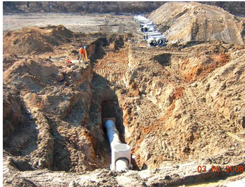
Sewer trench construction Image courtesy of Tetra Tech
